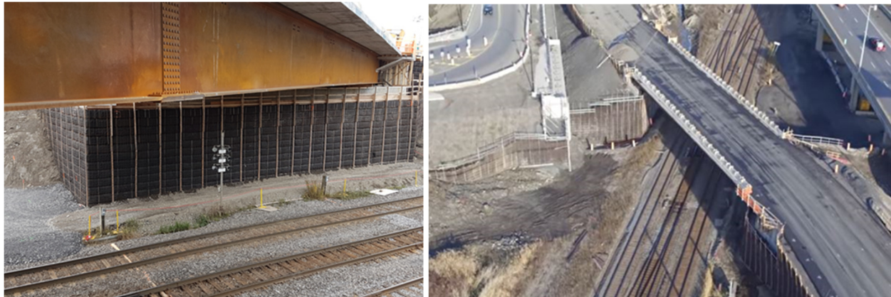
Figure 11: Temporary “true” bridge abutment with wire mesh facing
