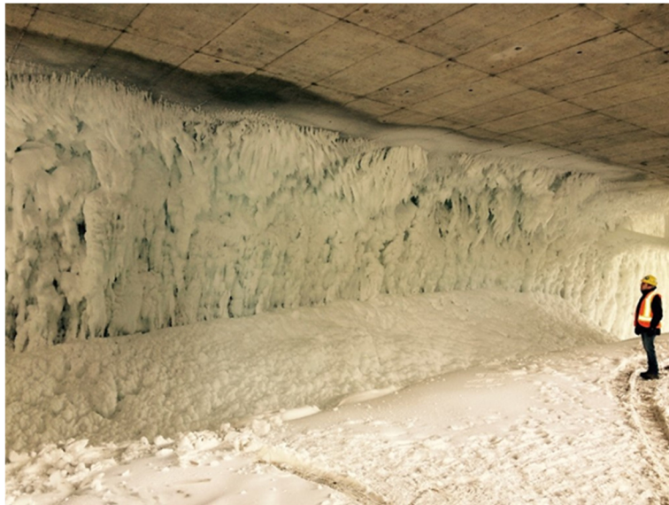
Figure 14: Icing protection of temporary MSE wall facing
