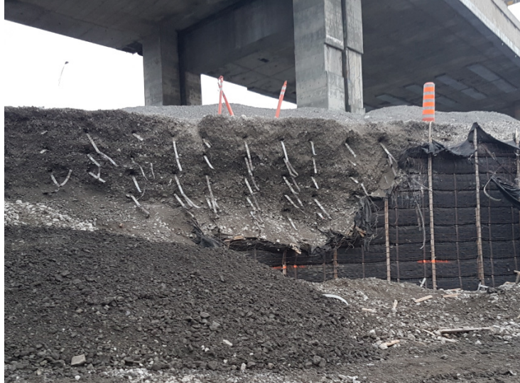
Figure 15: Dismantling of temporary MSE ramp
