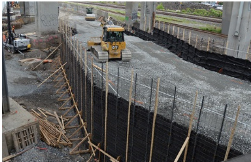
Figure 6: Temporary ramp fit in between existing structures' piles.
