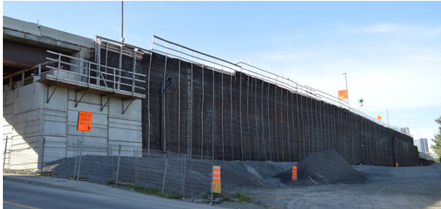
Figure 10: Temporary “true” bridge abutment with concrete panel facing
