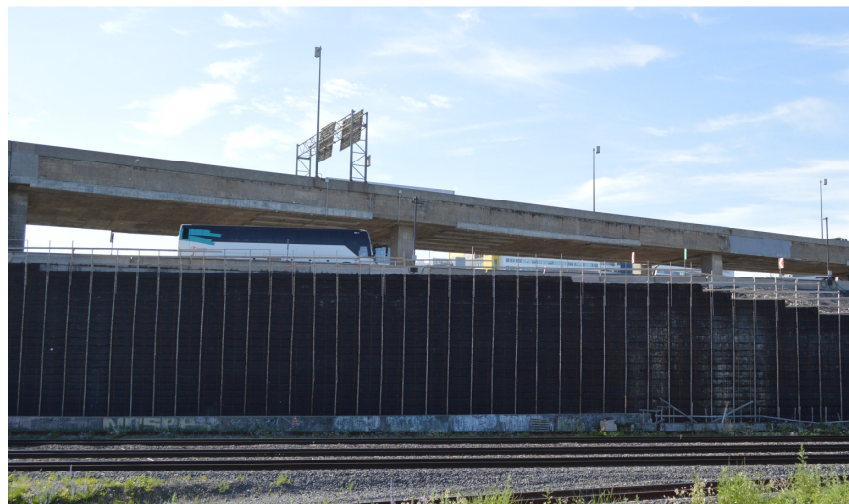
Figure 7: Tall temporary access road.
